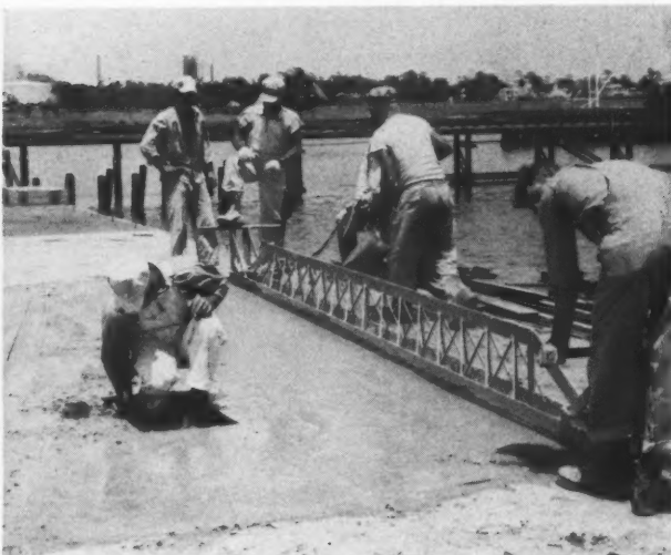
STURDY FLATBOAT chugs busily between dock structure and shore, delivering bucketsful of concrete and returning to mixer for refills. Workmen (below) smooth out concrete after it is poured on the deck.
